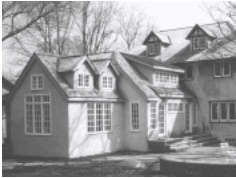
the new rear addition of the home
