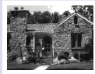
This charming 1930s stone cottage was torn down in 2003. It had irreplaceable character.
