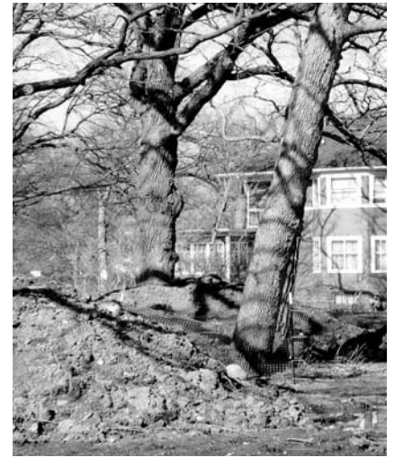
When the home at 682 Hillside was demolished for a much larger home, a vast number of pre-settlement Oaks were removed from the lot. The so called “protected” ancient Oaks, (above) had clay-laden construction debris heaped around their root zones and will most likely die.
